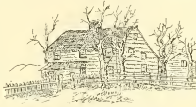
SAYRE HOUSE, SOUTHAMPTON. Recently Condemned.
