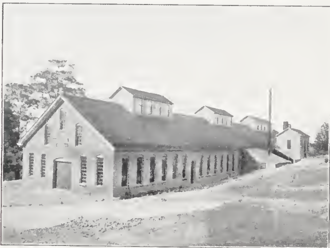
INDUSTRIAL BUILDINGS, MORRISTOWN COLLEGE
