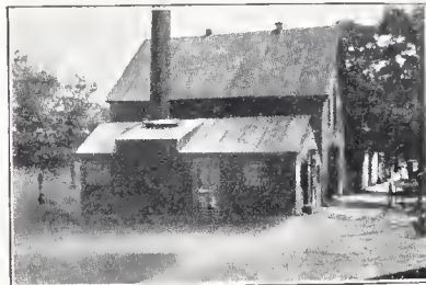
BOILER ROOM AND MACHINE SHOP
