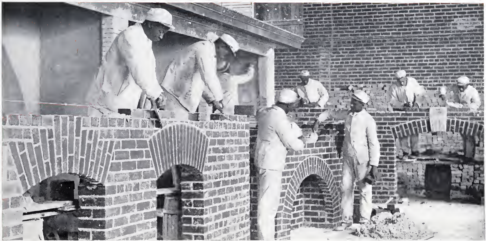
BRICK LAYING DEPARTMENT, HAMPTON INSTITUTE, HAMPTON, VA.
