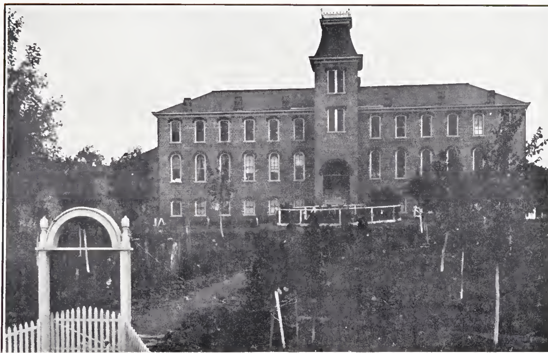
MAIN BUILDING, SWIFT MEMORIAL COLLEGE, ROGERSVILLE, TENN.
