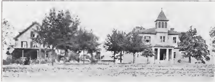
GIRLS' DORMITORY AND SCHOOL BUILDING
