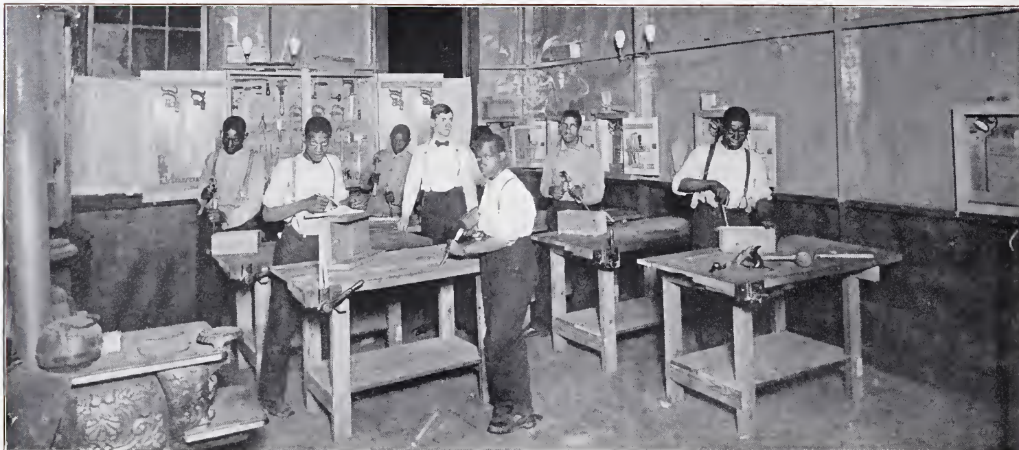
PRESTON STREET CARPENTER SHOP, LOUISVILLE KY.
