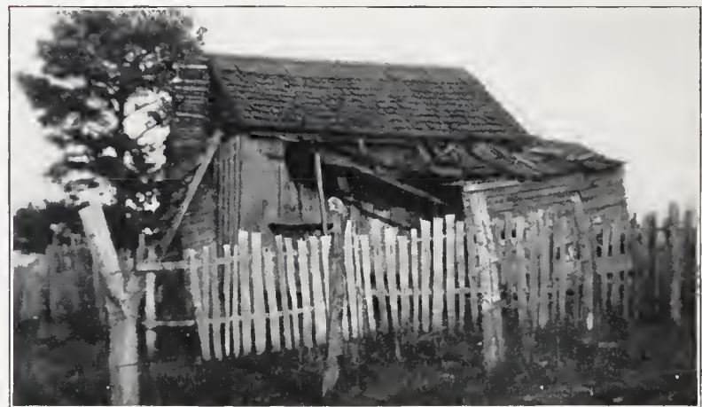
CABIN WHERE CALHOUN WAS STARTED, 1892
