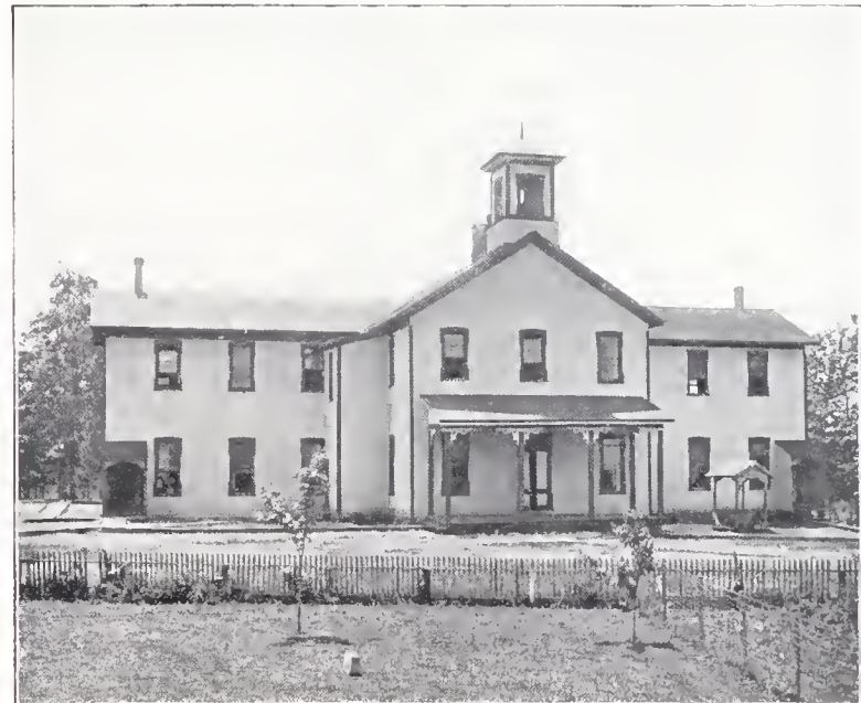
THYNE INSTITUTE SCHOOL BUILDING
