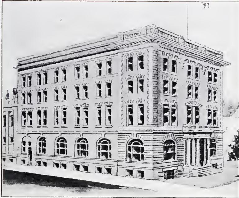
Y. M. C. A. BUILDING FOR THE COLORED MEN OF WASHINGTON, D. C.
