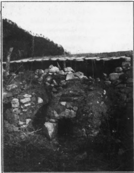
BLAST-FURNACE FOR PRODUCING MATTE.
