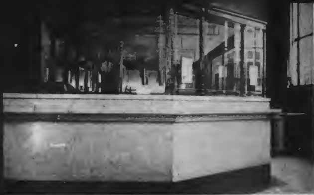
Before: View of the old-fashioned high plate glass counter screen with its ornate metal grills, dividing main tellers section
