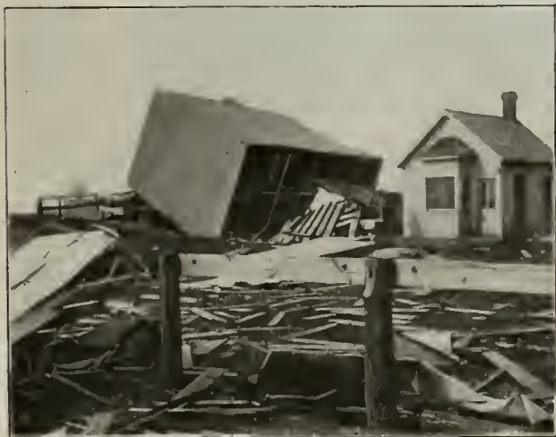
WHITE HEATH ELEVATOR AFTER THE CYCLONE.
