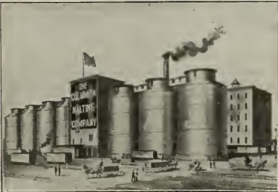
1,000,000 BU. FIREPROOF ELEVATOR.
