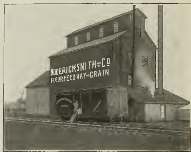
ELEVATOR OF R. SMITH & CO., DULUTH.
