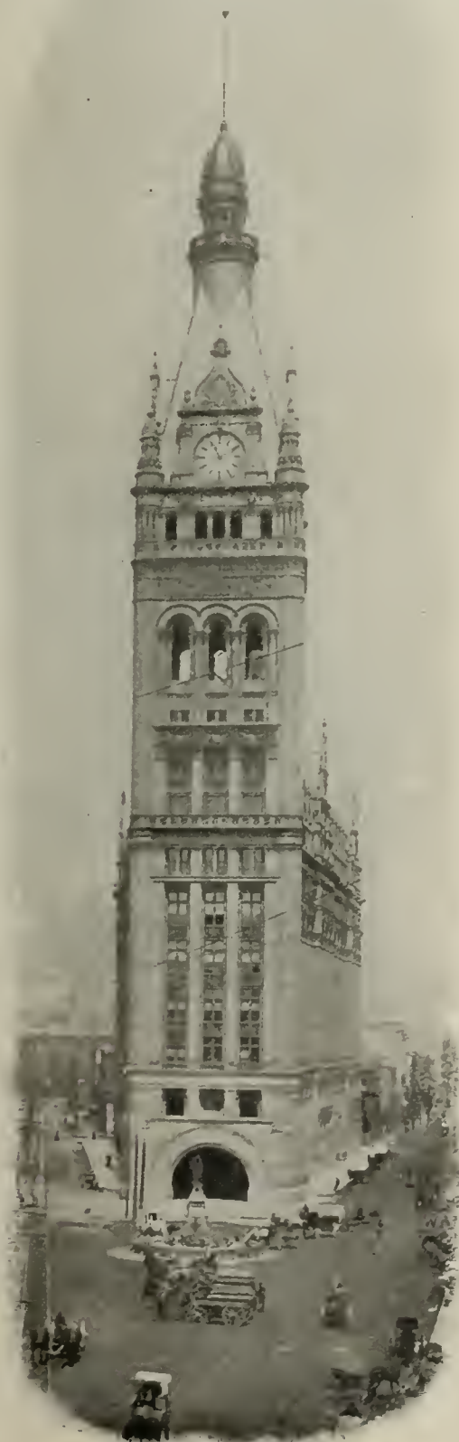
CITY HALL, MILWAUKEE.
