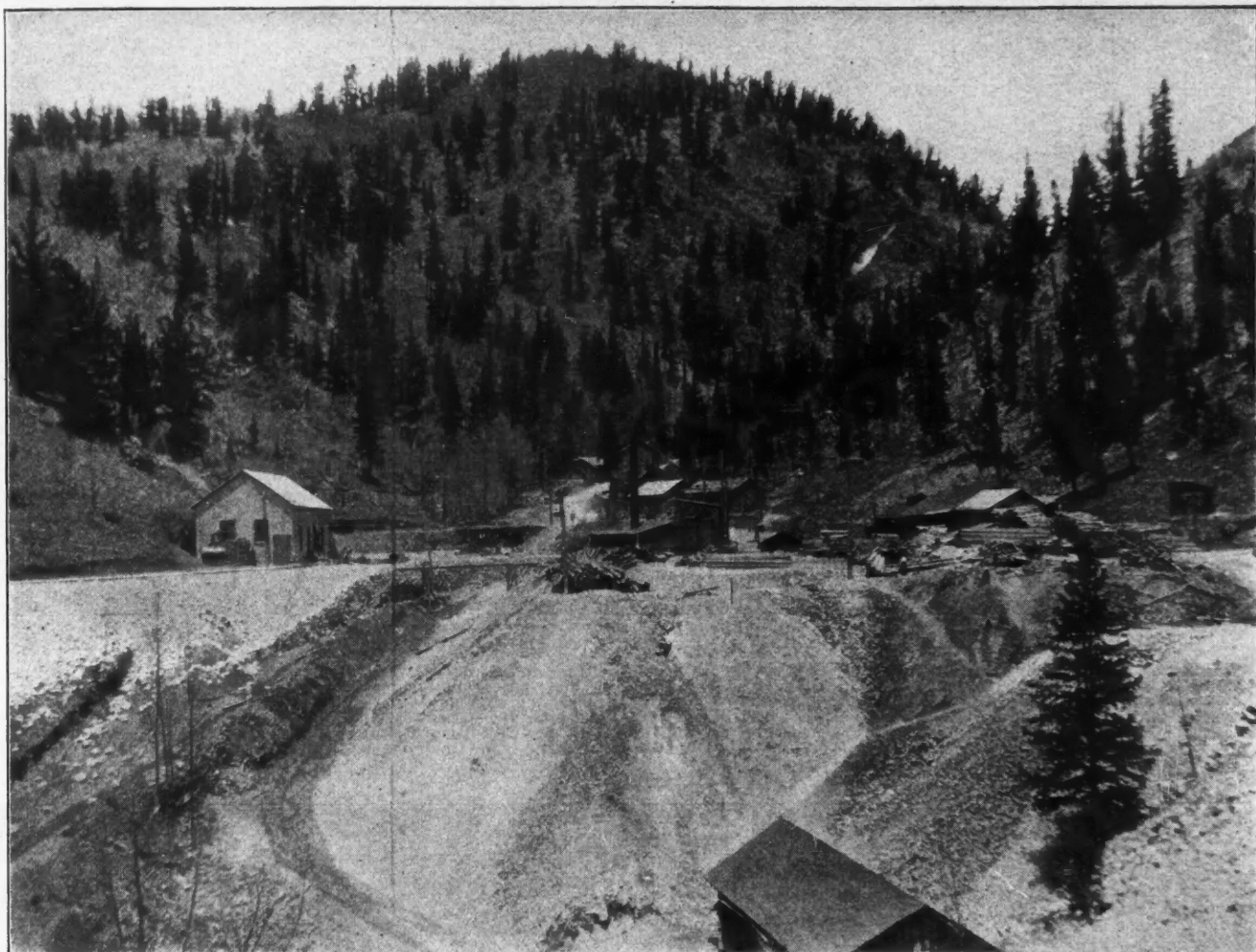
BUILDINGS AND SURFACE PLANT, RAWLEY MINING CO.
