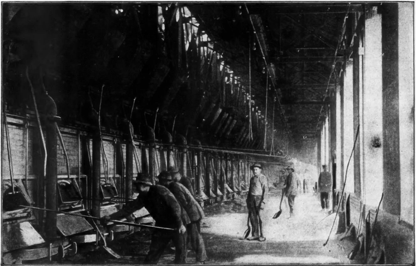
INTERIOR VIEW OF FURNACE BUILDING, EAST PLANT, NEW JERSEY ZINC CO., PALMERTON, PENN.
