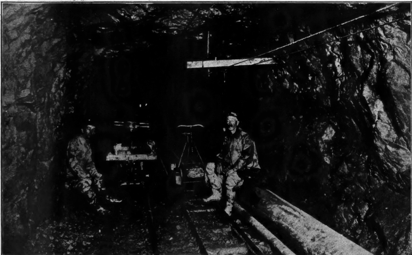
MAIN HAULAGE TUNNEL ON 1200-FT. LEVEL OF RAWLEY MINE, BONANZA, COLO.
