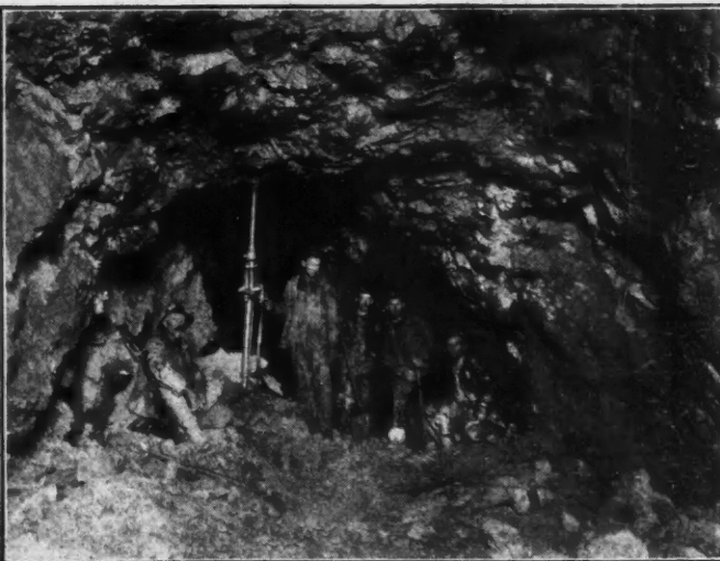
VIEW IN SOUTH STOPE ON THE 1200-FT. LEVEL
