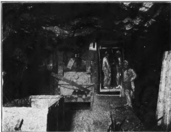
STATIONS OF MAIN RAISE AT THE 1050-FT. LEVEL
